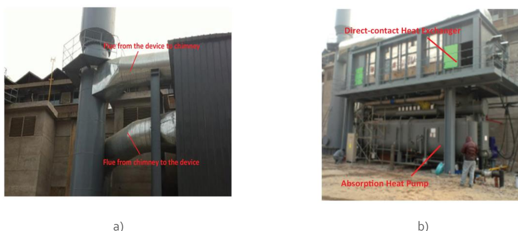
Figure 32: a) Connection between the chimney and the WHR system; b) WHR system composed by the direct-contact condensing HE and the AHP.
