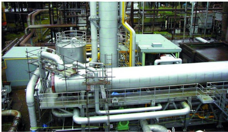
Figure 121: Photo of the low temperature 3.5 MWe Kalina power plant installed in a steel industry (Kashima Steel Works) in Japan (Global Geothermal, 2019).
