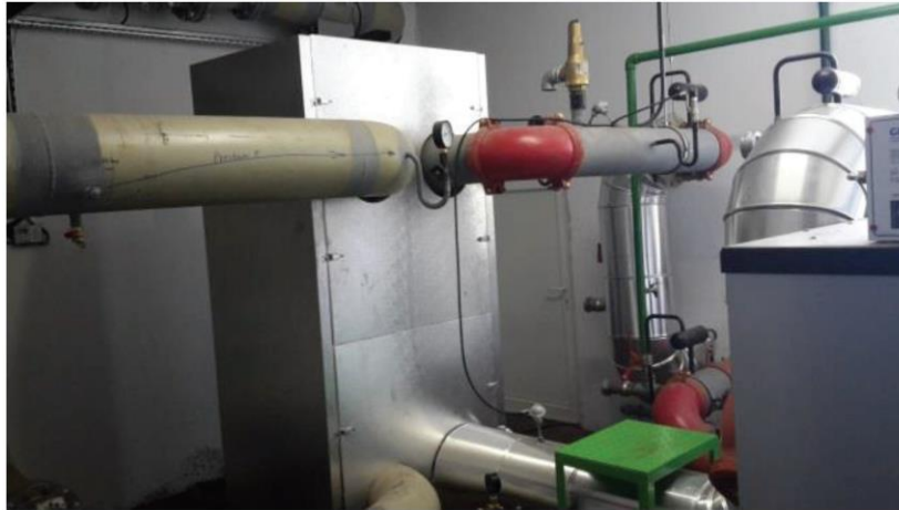
Figure 9: PHE (4.2 MW) for WHR from an EAF in a steel plant (Konovšek et al., 2017).
