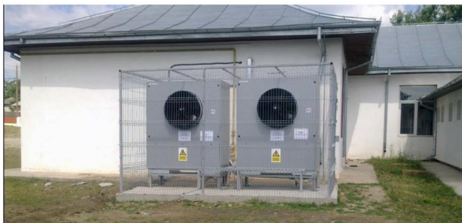
Figure 212: Photo of an ASHP for space and water heating installed in a school in Romania (Popa et al., 2016).
