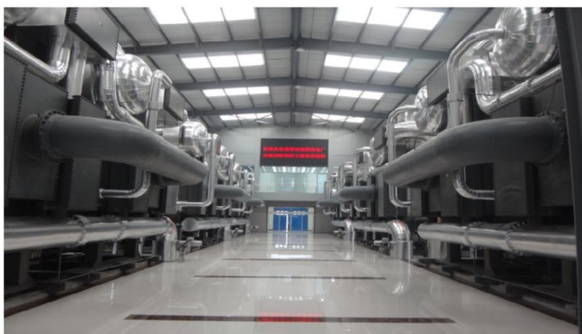
Figure 221: Large scale (290 MW t ) steam driven AHP for district heating in Lanzhou (China) (Z. Y. Xu et al., 2018).
