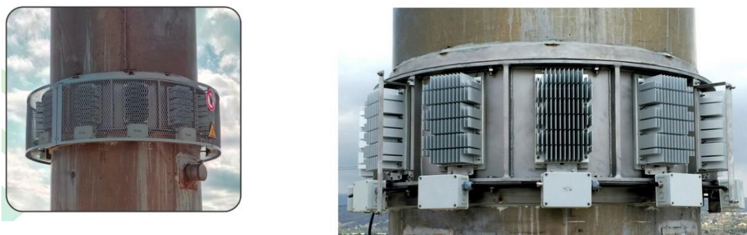
Figure 182: Examples of TEG systems installations in chimneys (AEInnova, 2019).
