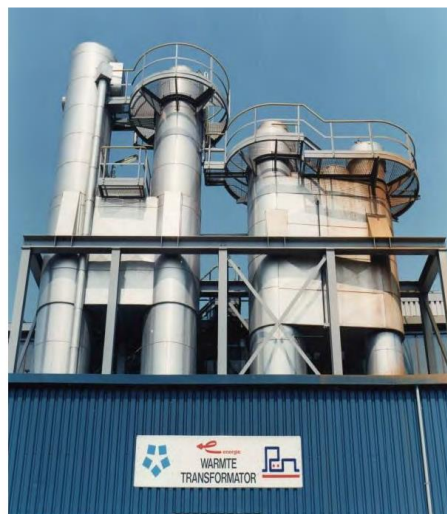
Figure 225: Heat transformer installed in the nineties in the Netherlands to upgrade the WH released in a hot rolling strip mill (IEA Task 35, 2014).
