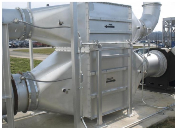
Figure 75: Gas-to-air HPHE ("Econotherm," 2020).
