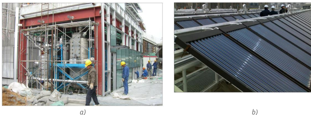
Figure 131: Solar thermal Kalina cycle demonstration plant built at EXPO 2010 Shanghai (China): a) construction of the power plant; b) evacuated solar collectors installed on the roof of the EXPO Pavilion (Wasabi Energy Limited, 2010).
