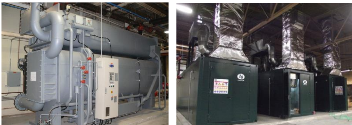
Figure 92: Absorption chiller Carrier and engines MWM in Simonds Plant (U.S. Department of Energy, 2017a).
