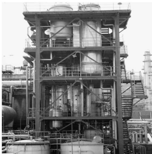
Figure 224: Single stage 5 MW AHT installed in a synthetic rubber plant (Xuehu Ma et al., 2003).
